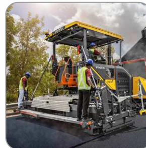
Road Construction Equipments
